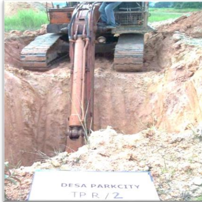
TRIAL / TEST PITS
