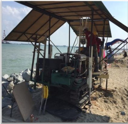
CONE PENETRATION TEST
